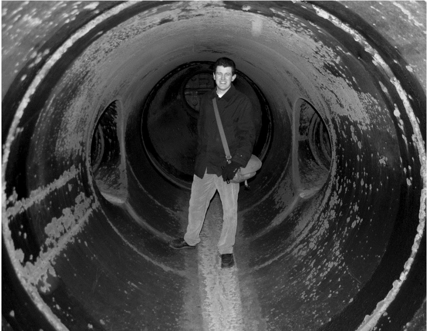
Figure 12. An urban explorer appreciates the acoustics inside the Halfway Pipe. 20110202
