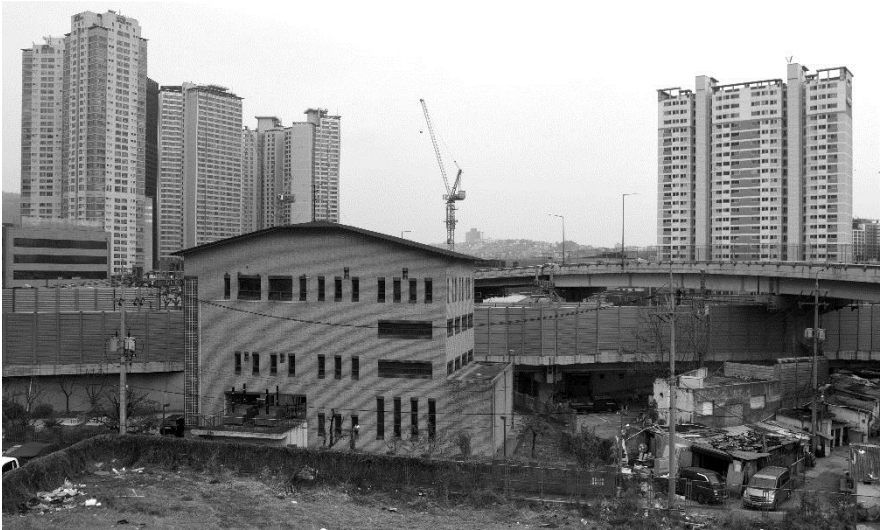
Figure 19. Munbae Pump Station is a large, plain facility. To its right is a small shantytown that backs onto Manchocheon. 20190421
