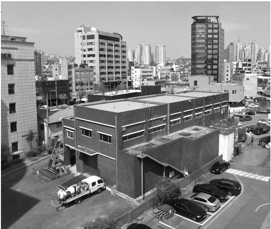
Figure 13. Wonhyo Pump Station is a large brick building in the alleys of Yongsan Electronics Market. It is unlabeled except for one plaque not easily visible from off property. 20190419
