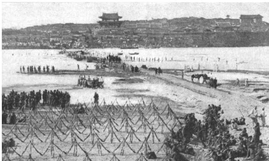
The pontoon bridge being built at Pyongyang. 53
