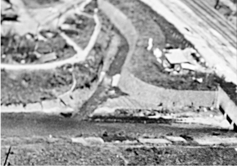
Figure 16. Compare the shape of the slots under the bridge in the lower right corner here to the photos below and on the previous page. Blowup from Fig. 6. Courtesy of Yongsan Legacy
