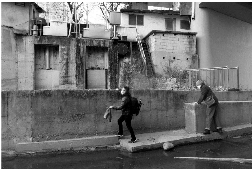
Figure 18. Two explorers hug the wall along the clearing north of the Gyeongui Line bridge. The catwalk and staircase lead into a shantytown, and the sluice gates lead to Munbae Pump Station. 20181222
