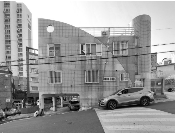
Figure 8. Another view of the 1997 Choryang-dong building in Figure 7. Its colors and architectural lines are reminiscent of the Art Deco resurgence in the 1980s, particularly those found at Miami Beach.
