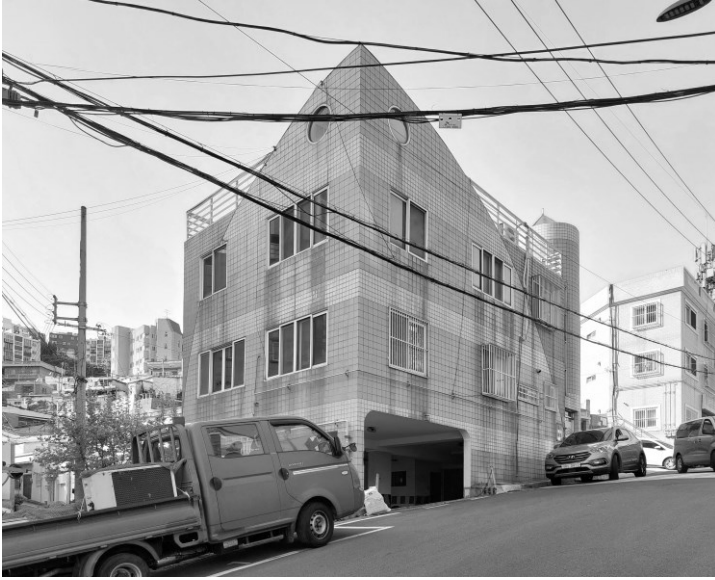
Figure 7. A three-story mixed-use building of sky blue, cream white, and azure tiles in Busan’s Choryang-dong appears to be a product of the reinterpreted Art Deco styling that came out of the 1980s and continued into the 1990s. The building dates to 1997.
