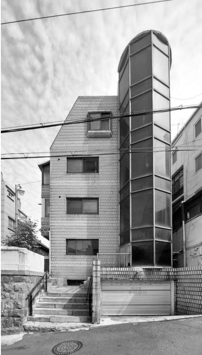
Figure 10. A mixed-use building in Huam-dong dating to 1992 is transitional in features and materials. It uses the modern bay windows and amber-gray glass common in the 1980s, but adapts curtain wall glass and the pastel blue and white colors popular in the 1990s.
