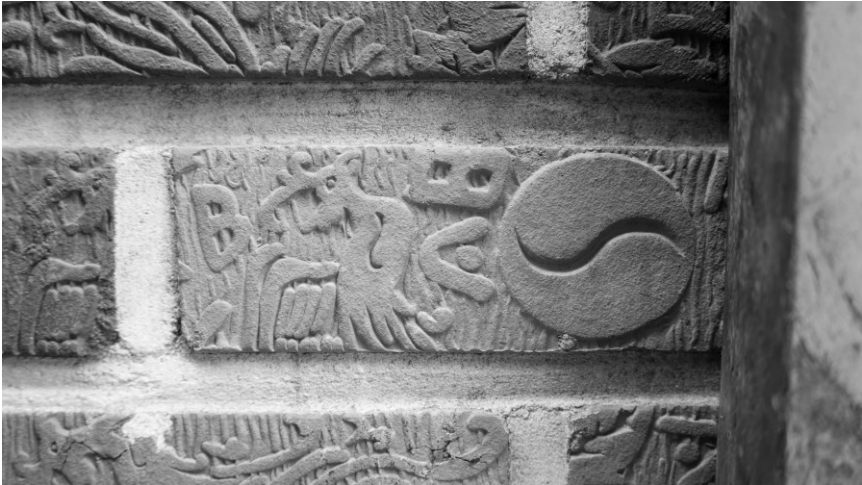
Figure 6. A red-brown, brickish-tile molded with nationalistic icons on a four-story multi-use building dating to 1995 in Yongsan-gu, Seoul. The building format is similar to the typical villa of the 1980s.
